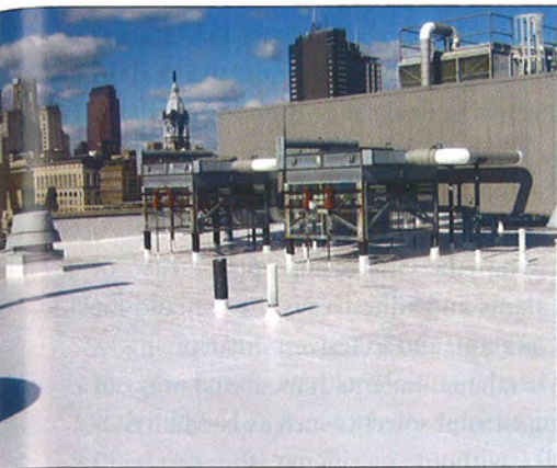
Urethane coatings that meet current emissivity and reflectivity requirements are becoming increasingly popular.
